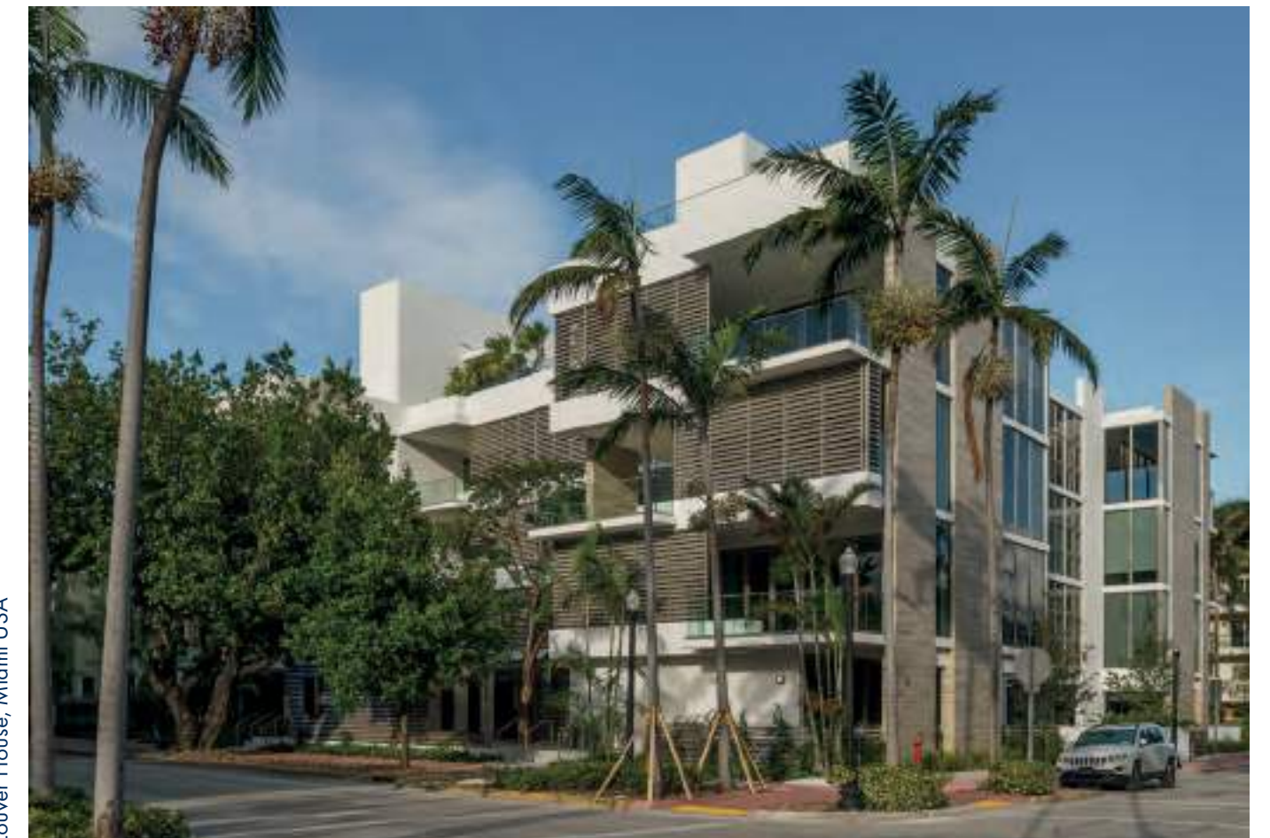
Louver House, Miami USA
